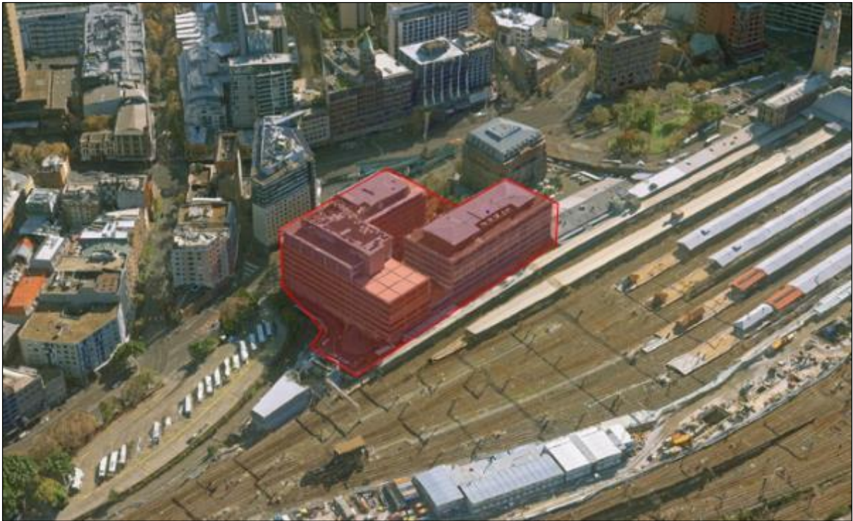
Figure 2: Oblique aerial of the subject site, looking north-west.
