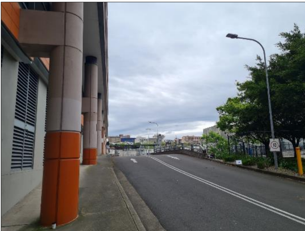
Figure 10: Existing vehicular access to basement from Lee Street, looking east.
