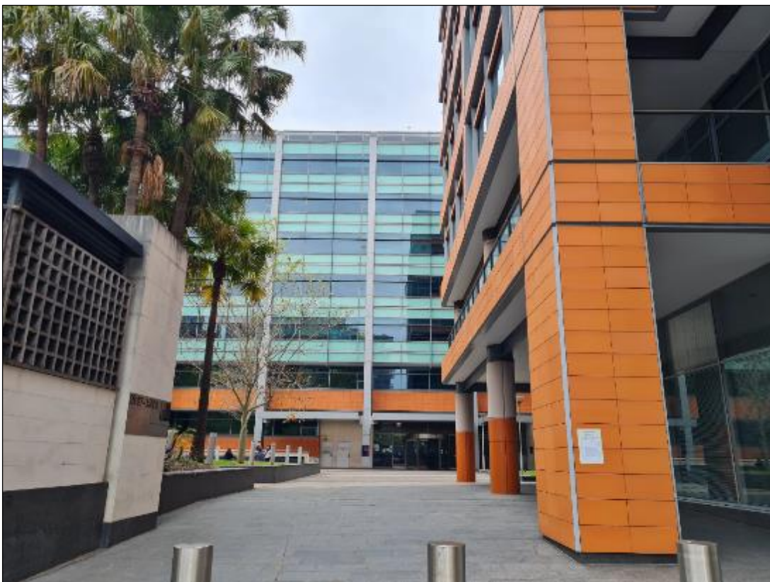
Figure 6: View and access into the site from Lee Street.
