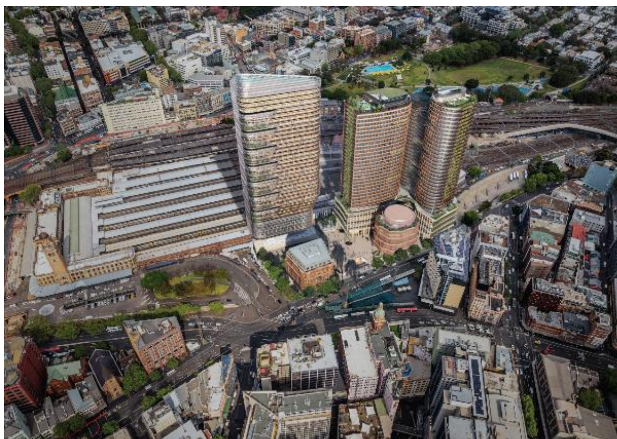
Figure 71: Oblique photomontage of the development and the relationship of the red colour palette of the tower and Connector building with other red masonry buildings in the locality.
